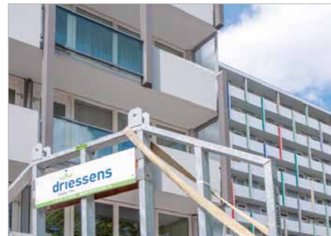
A future-oriented market: Facade renovation
