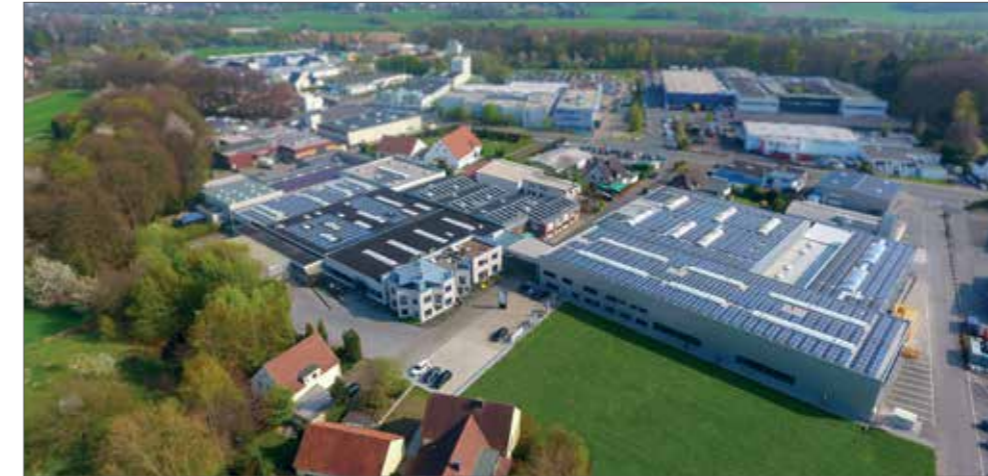
Company HQ in Brake, in the outskirts of Bielefeld, with 7 production halls and a total production area of 12,000 m 2 .
